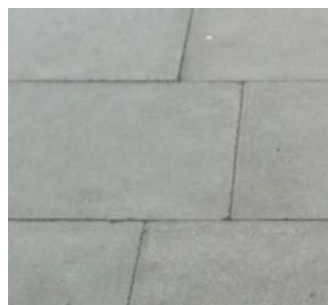
Concrete flag pavers
