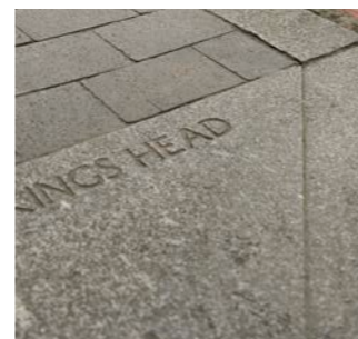
Granite kerbs and quadrants
